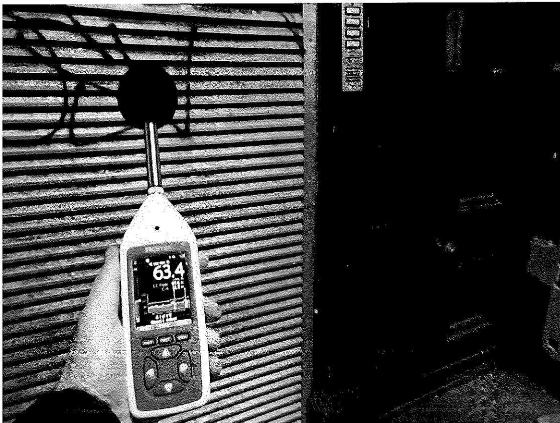
Figure 4: Plant noise at 1m.
